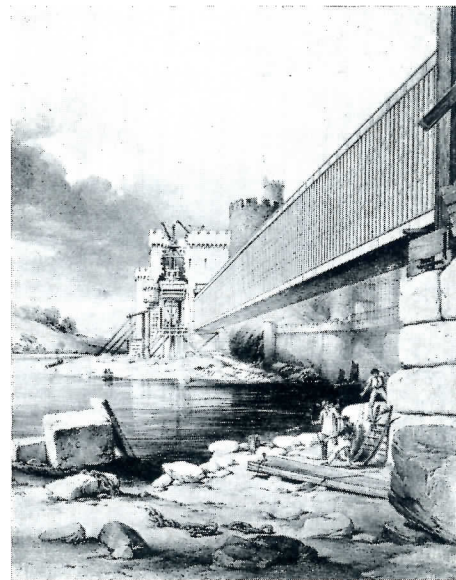
Building the Conway Bridge.
