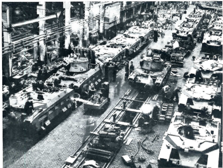
Erecting "Matilda" Tanks during the War.
