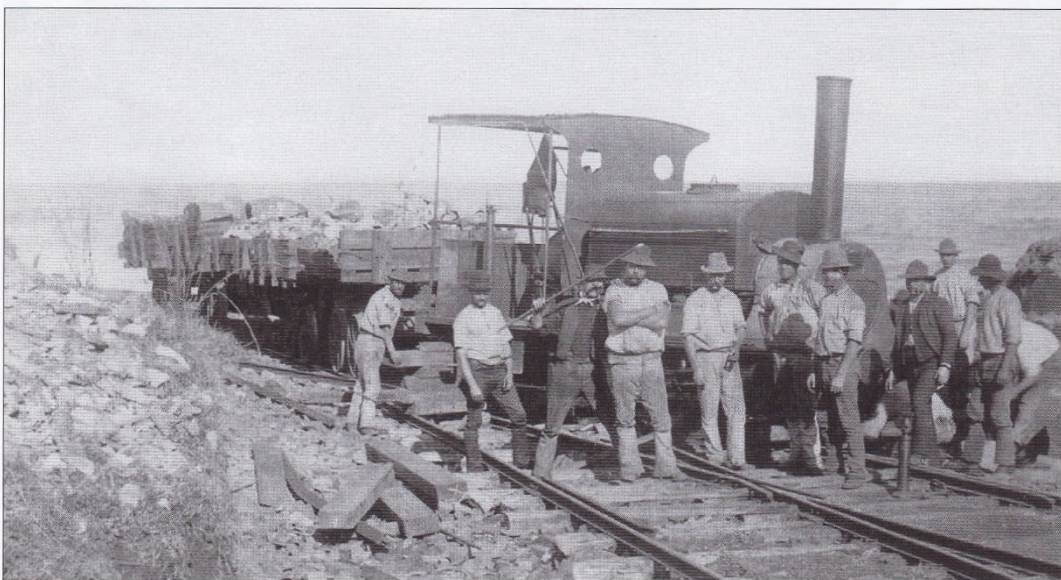
An unidentified 0-4-0 saddle tank at Harrington in some trouble on a stone train for breakwater construction at the mouth of the Manning River. (Imperial Studio, Bruce Macdonald collection)
