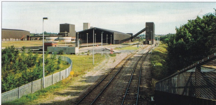
A deserted Asfordby Mine in August 1997.
