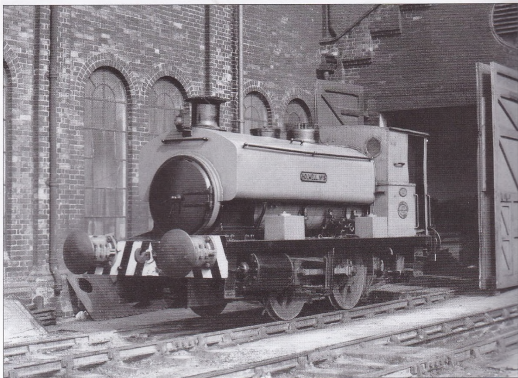
HOLWELL No.18 (Andrew Barclay 1791/1923) had been recently repainted and was pulled out of the Holwell Ironworks shed for a photograph on 28th March 1969. Note the distinctive heavy buffers that were a feature of the locomotives at Holwell. (Cliff Shepherd photograph)
