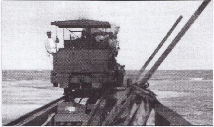
The Clarence River locomotive propels a loaded tip wagon on timber staging erected for training wall construction c.1896. (Clarence Valley Historical Society)
