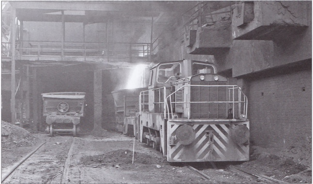
Number 250 (Thomas Hill 252V) waits whilst slag is tapped from one of Ravenscraig's blast furnaces on 18th July 1985. The remains of a Hunslet 0-4-0 diesel hydraulic is placed ahead of the leading slag ladle to protect the locomotive. A more colourful view of this scene can be found on the rear cover of RECORD 245. (Martin Shill photograph)
