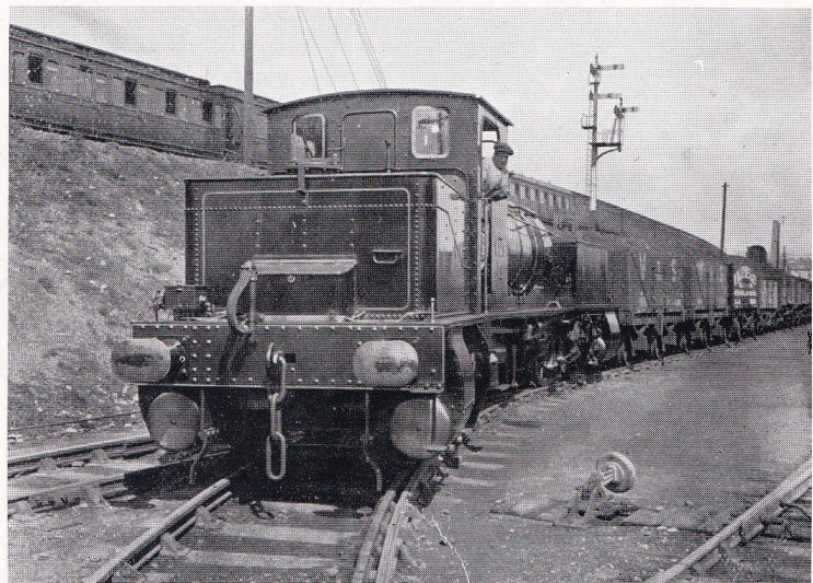
“Garratt” Locomotive entering 97 feet radius curve at the Hafod Copper Mills.
